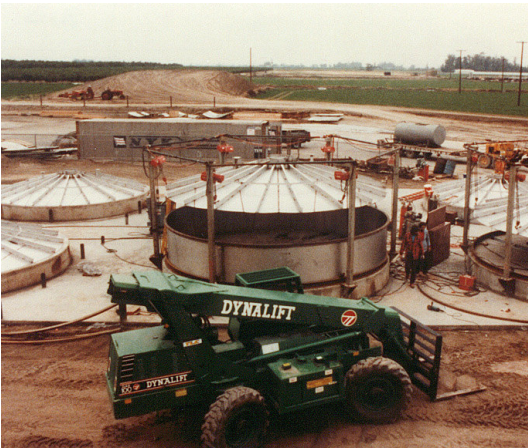
A series of tanks under construction.
