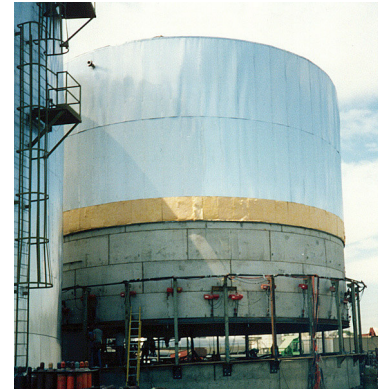
A vertical, cylindrical storage tank almost completed.
